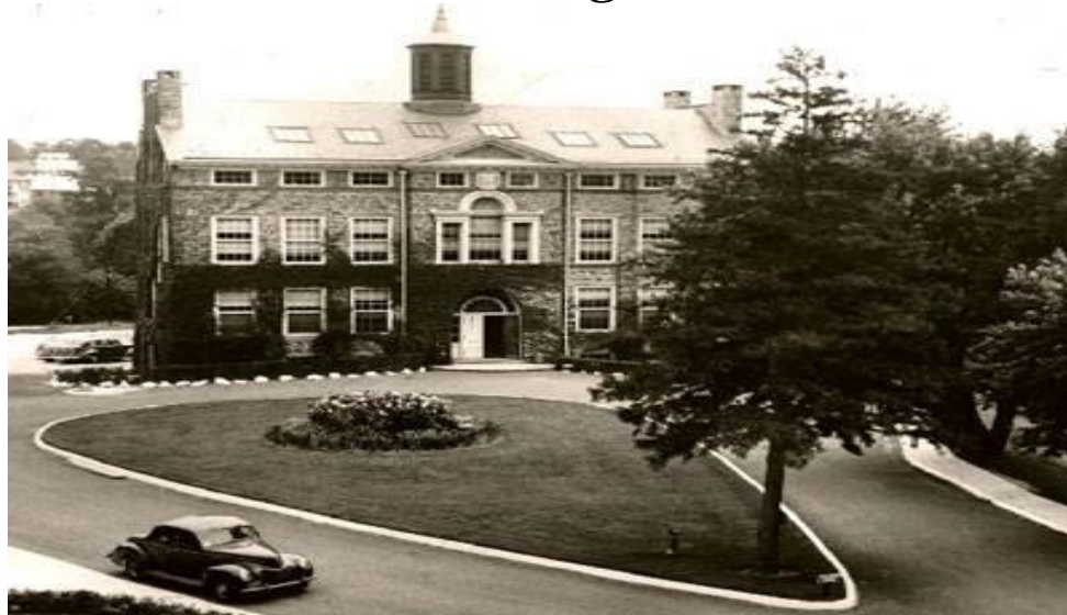
Carnegie Hall, the oldest classroom building on campus ( Built in 1919 )
